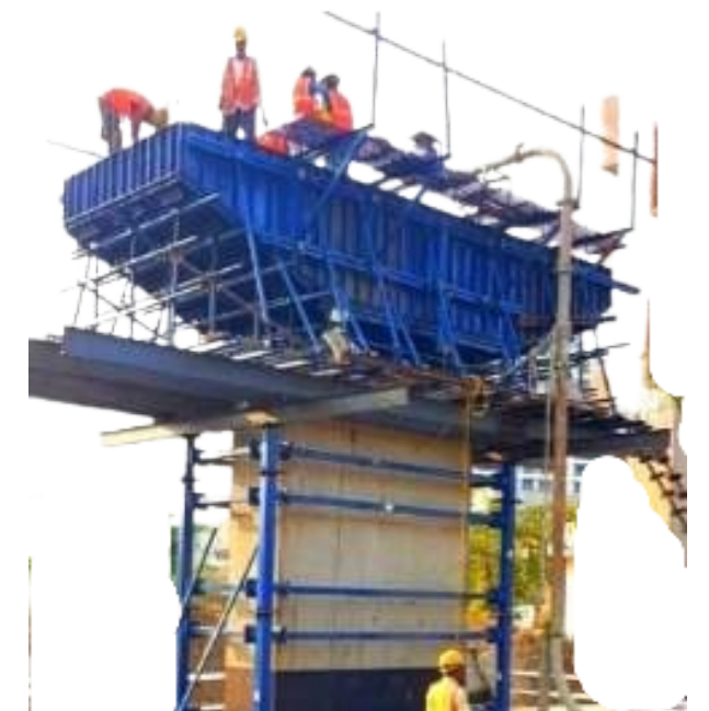
Pier Cap Formwork
